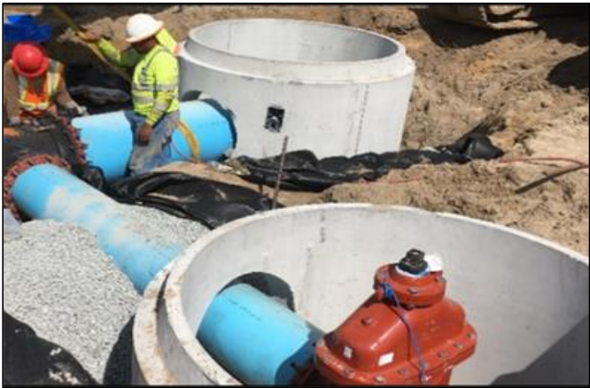
24" Water Main and Valve Installation SAVANNAH savannahga.gov
