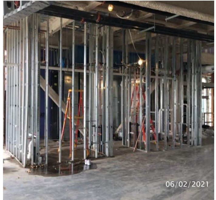
Overlook Quad 3 - Crews installing framing for Restrooms near Stairwell #3 - Looking South.
