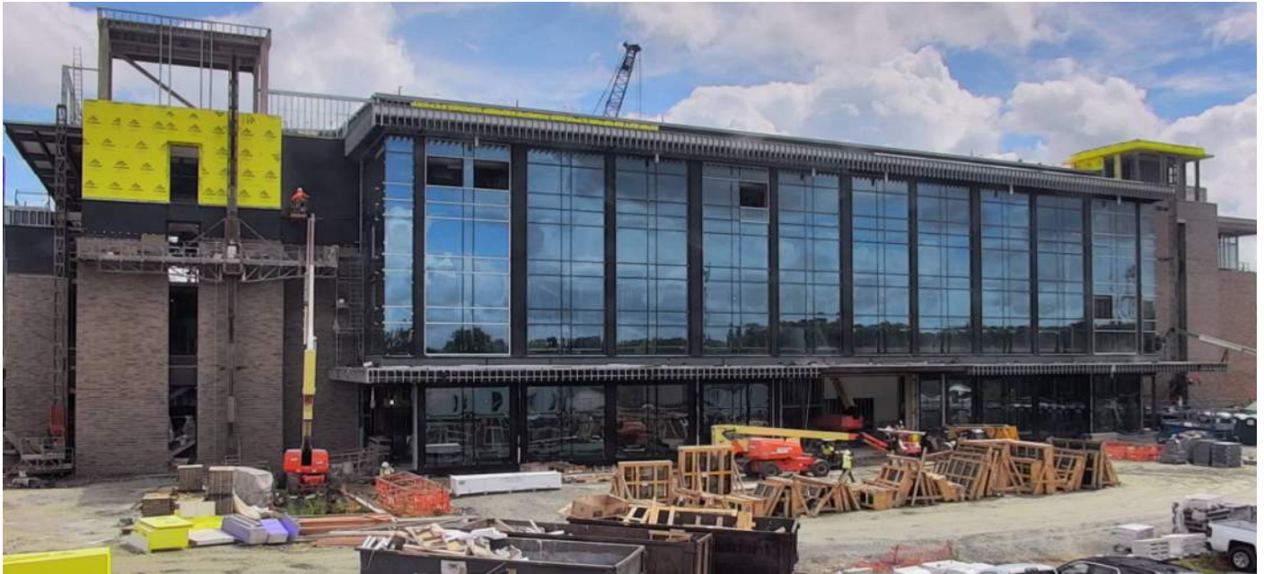
Southern Elevation looking Northeast.
