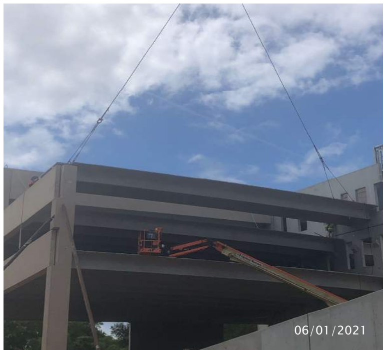
Parking Garage - Crews continue with precast erection - Looking East.
