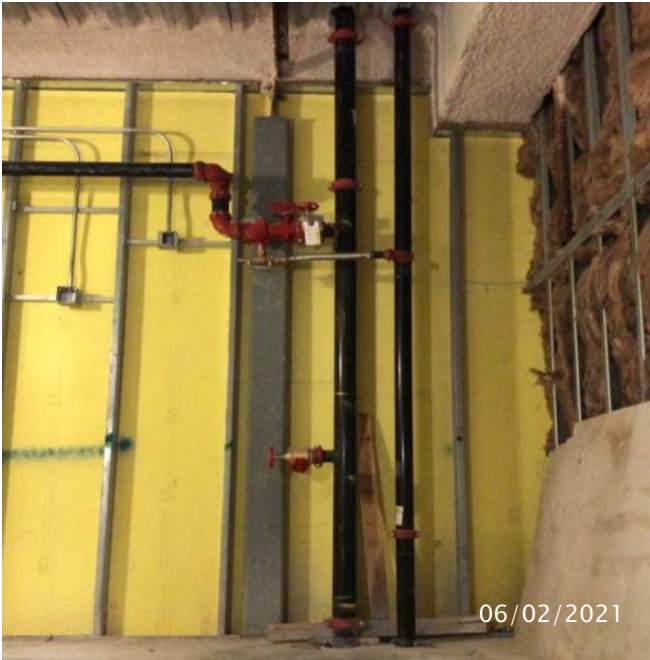
Northeast Stairwell - Fire protection risers installed in stairwells – Looking West.
