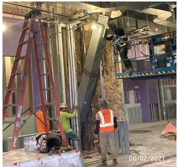
Concourse Quad 2 - Crews removing temporary steel in North Bar Area - looking Northeast.
