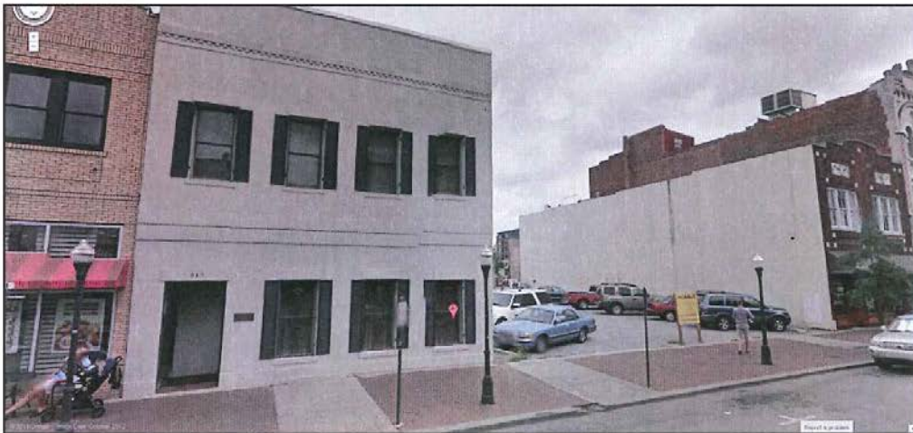
240 W. Broughton St., comprised of existing building and vacant lot.
