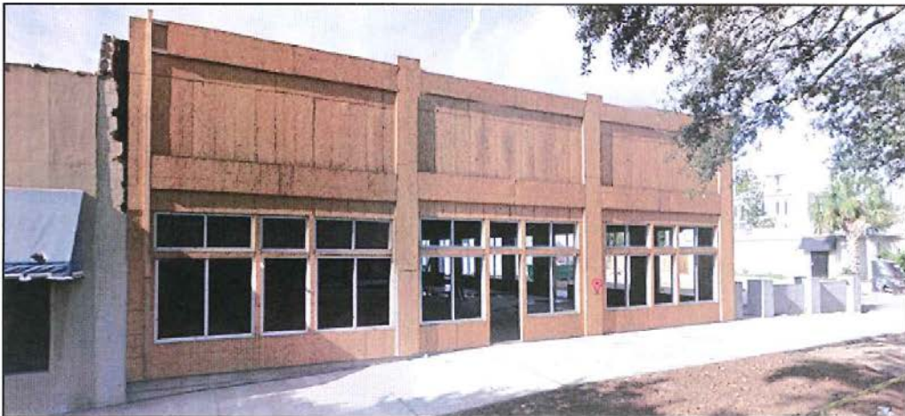
Front facade of 535 E. Liberty Street.
